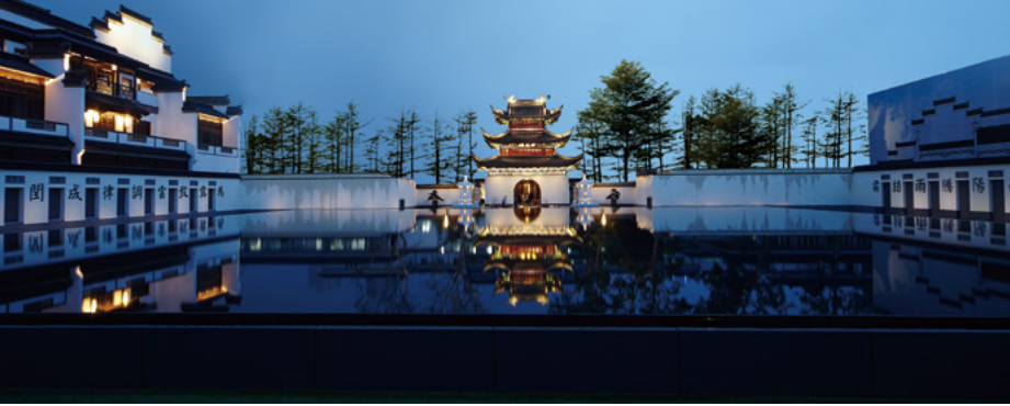
Building Facade & Landscape Lighting
